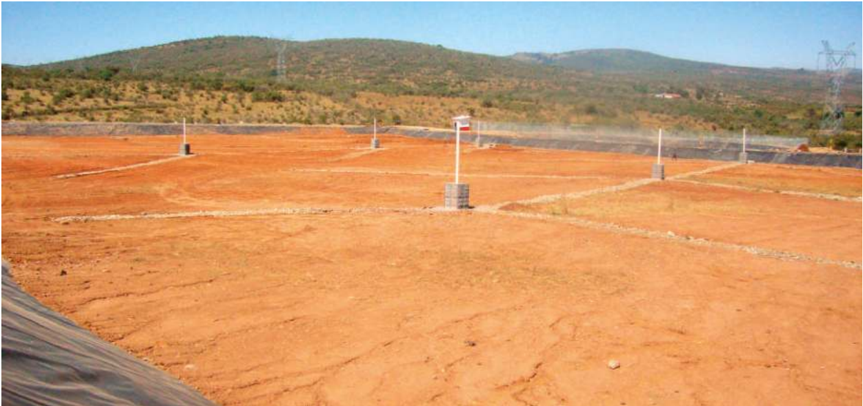
Relleno sanitario intermunicipal 2012
